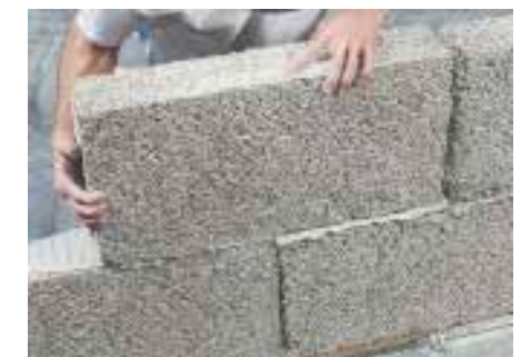
HempCrete - woody inner fibres of Hemp plant bound with Lime
