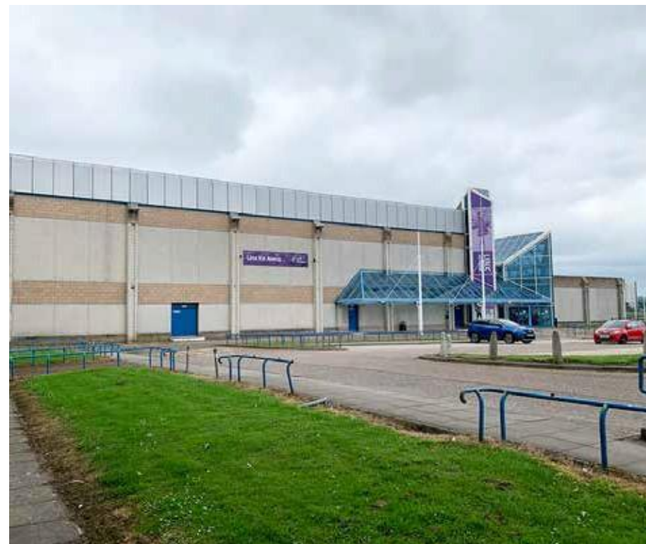
Existing Entrance and external facade
