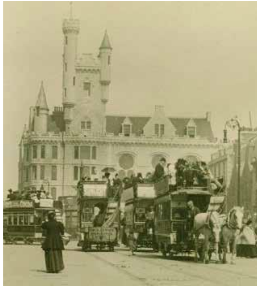
Tram Transport Hub at Castlegate
