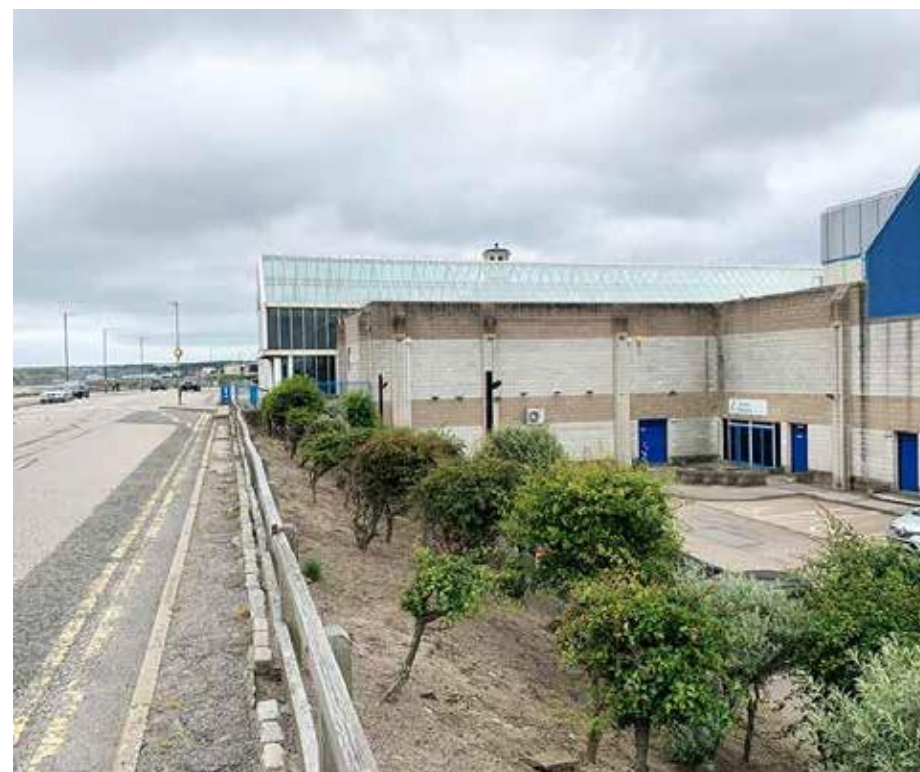
Existing Entrance and external facade
